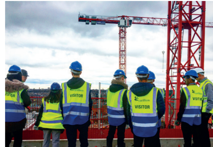
Work experience students on site at the Midlands Metropolitan Hospital
